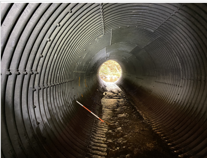
Barrel from Upstream End with Southern Wall Deformation
