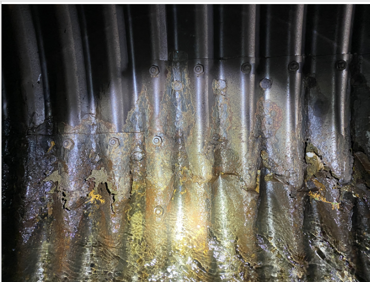
Perforations / Crushing on Southern Side of Panel #4 from the Downstream End
