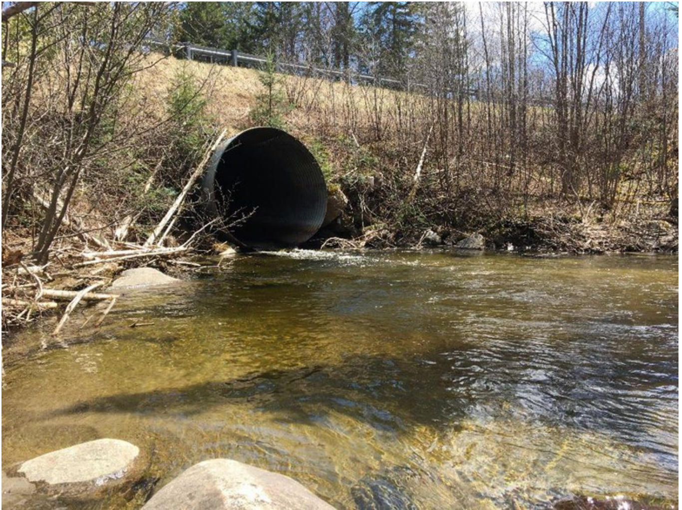
Outlet and scour pool (Inspection photo 2020)
