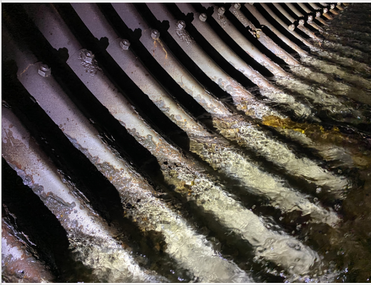
Southern Wall Perforations at Panel #7 from Downstream End
