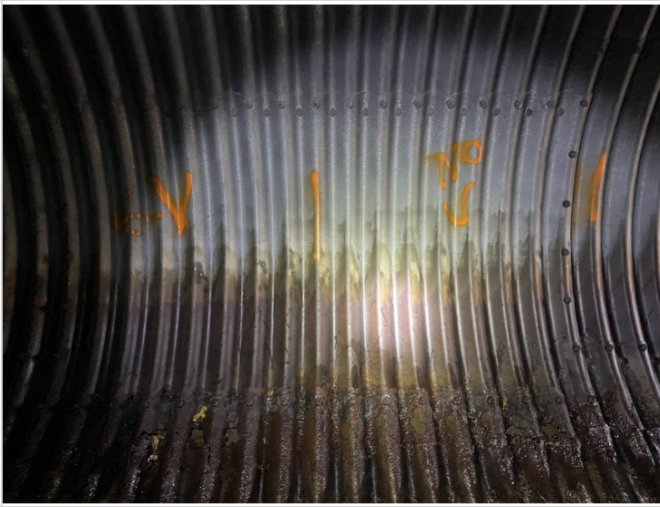
No Voids Present in Downstream Section of Panel #4 from Downstream End
