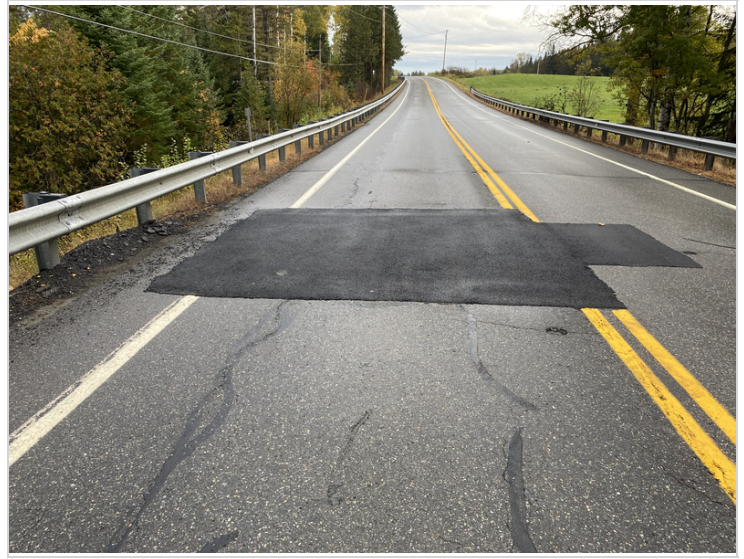
Asphalt Patch Over Downstream End
