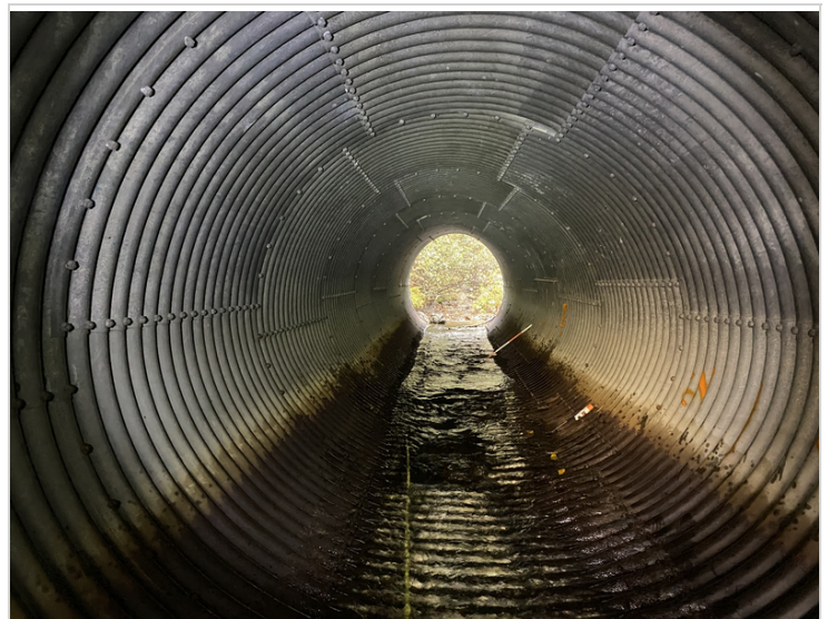
Barrel from Downstream End with Southern Wall Deformation
