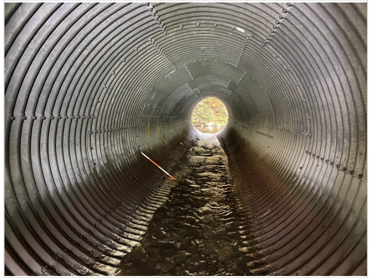
Barrel from Upstream End with Southern Wall Deformation
