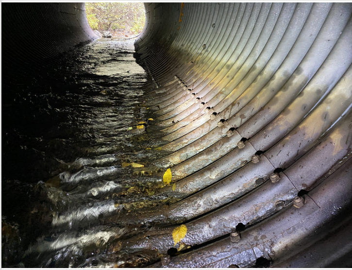
Panel #4 from Downstream End with Significant Bending on Downstream Portion and Large Perforations
