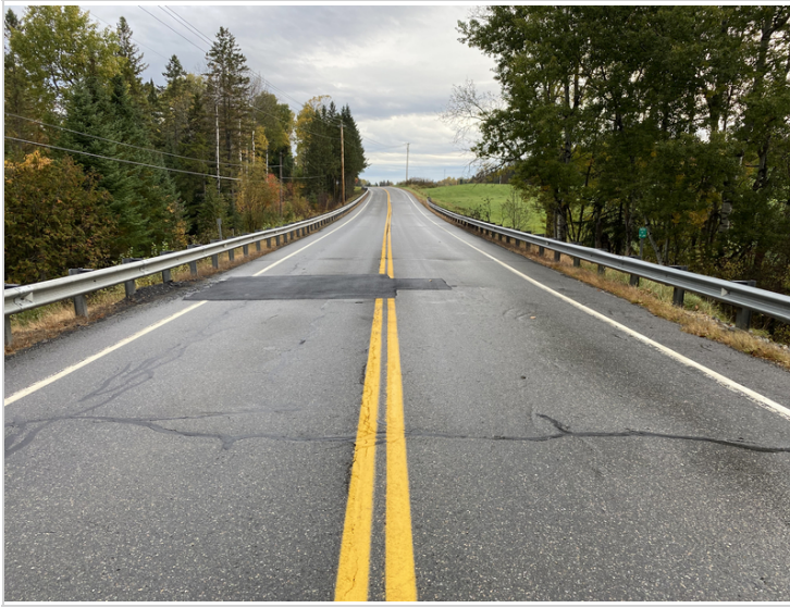
Asphalt Patch over Downstream End of Structure
