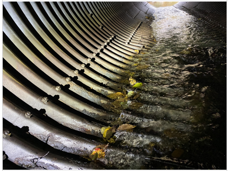
Perforations on Panel #5 from Downstream End on Southern End
